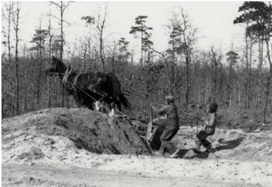
A vintage style of bunker creation in evidence at Pine Needles, North Carolina
